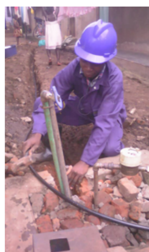
Ronald doing practical work in his plumbing internship
